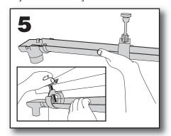
Place the gutter and clamps to the roof edge so gutter is suitably positioned, supporting the gutter as needed whilst nipping up the brackets enough to secure the gutter - **do not overtighten**.
